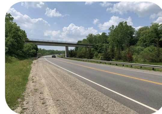
Highway 3 east of CNR Subway looking west.
